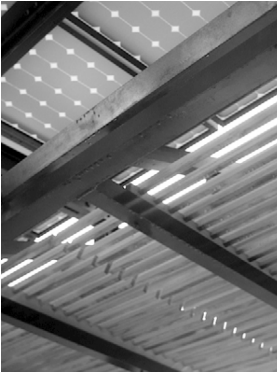
Fig. 1. Material Detail: Screen Door, Aluminum Frame and Photovoltaic panels (photo by Mark McGlothlin)
