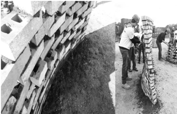
Figure 5: Examples of Folded and Curved Single Wythe Masonry Walls
