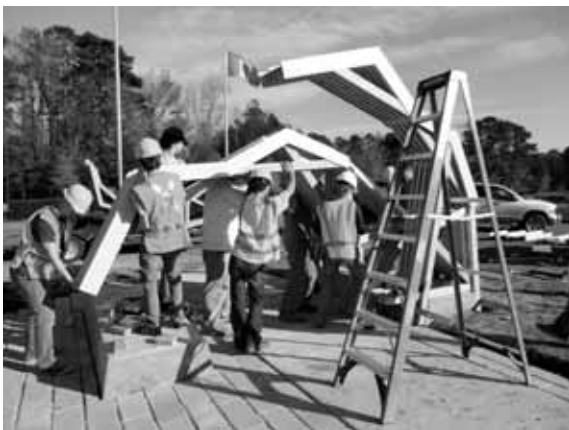
Fig. 1. Assembly of the Philadelphia, MS bus shelter. 6
