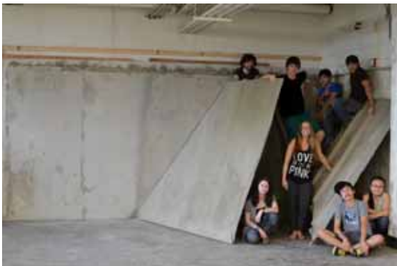
Fig. 9. Thin shell concrete folded out. Students: V. Bui, C. Canfield, J. Costello, J. P. Lauricella, C. Narvaez, J. Salton, H. Tanner, E. Zeffiro. Photograph by the student group.
