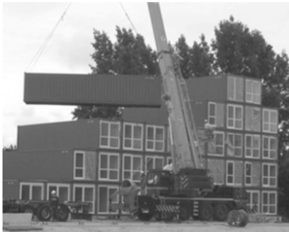
Fig. 7 – Stacking Containers by Crane
