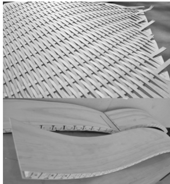
Fig. 11. CNC Zip-joint and woven rain screen
