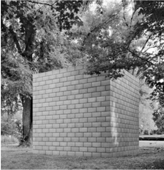
Fig. 1. "Cube" is built with 20 courses, each course consists of 10, respectively 11, full-size blocks and visible from all four sides (Image by Zellweger Park)
