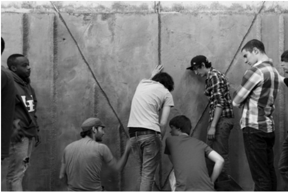
Fig. 8. Thin shell concrete cast against the studio walls with planned fold and reinforcement creases. Students: V. Bui, C. Canfield, J. Costello, J. P. Lauricella, C. Narvaez, J. Salton, H. Tanner, E. Zeffiro. Photograph: G. Rafailidis.
