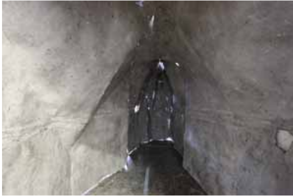
Fig. 12. Folded paper pulp thin shell.. Photograph: G.Rafailidis.
