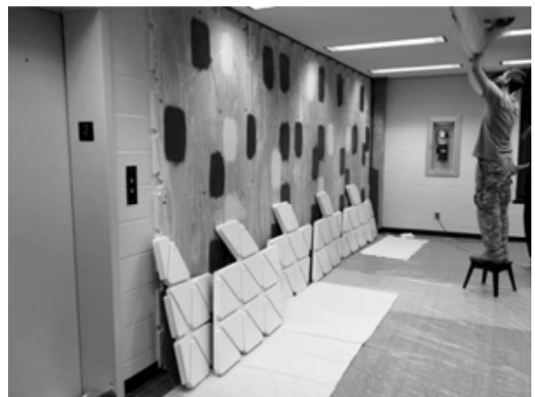
Fig. 13. Installation of the Plug-in Wall
